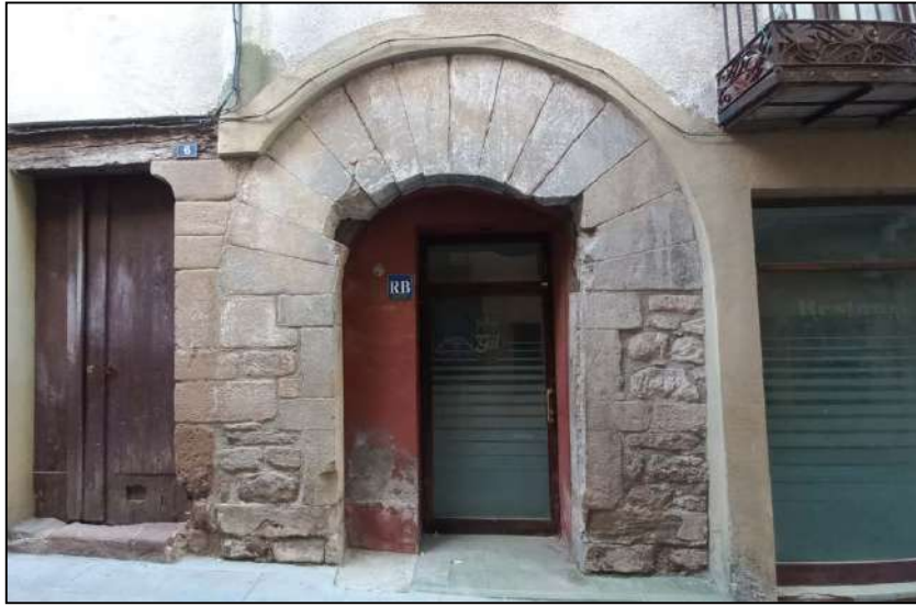
Fig. 14. Vista de la porta adovellada del carrer Major, 4.
