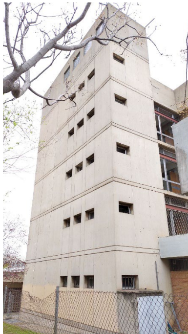
Torre tram C-D-A
