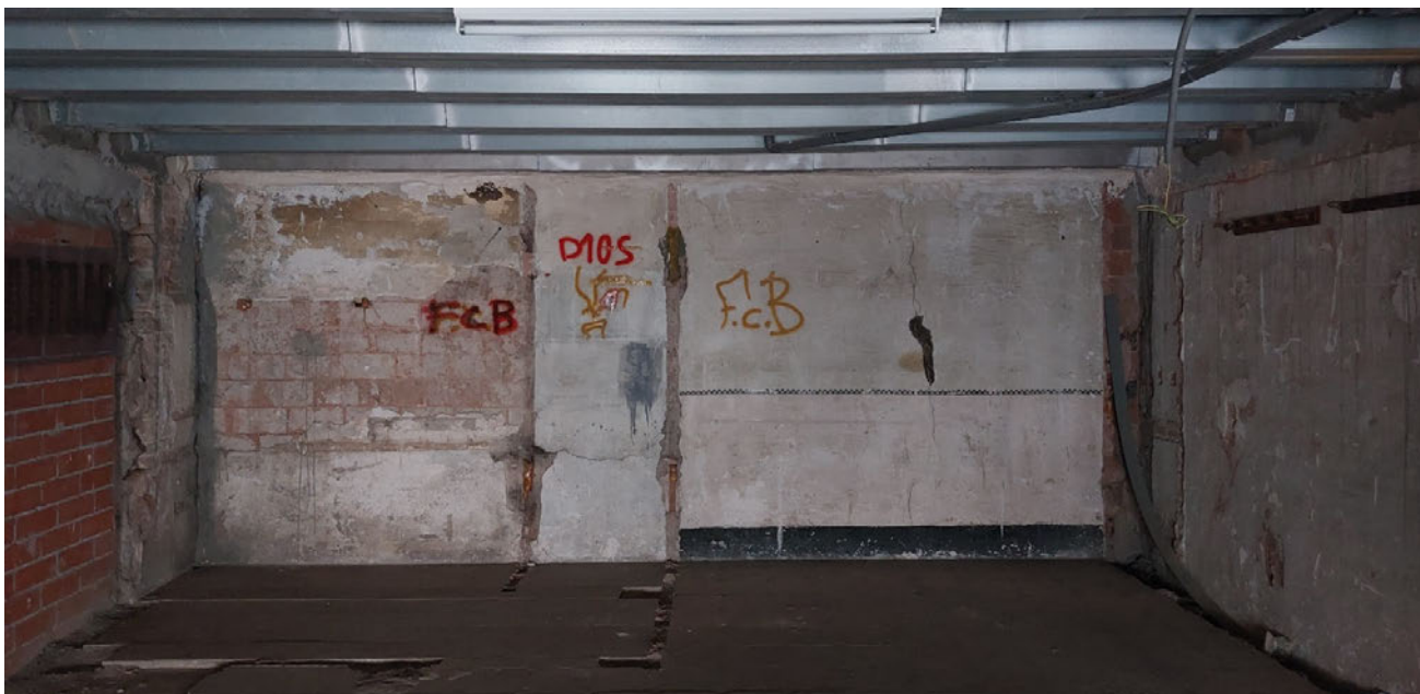
PA- Parament interior mitgera
