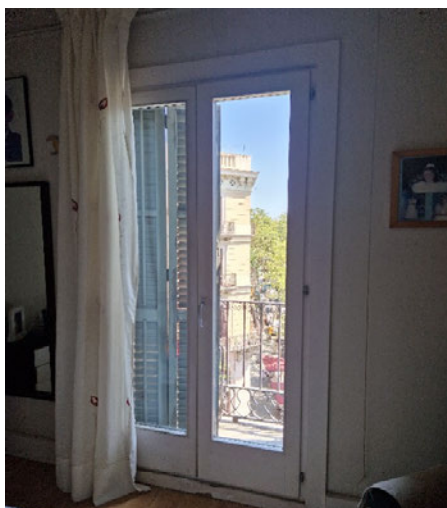
P4- Fusteries noves (interior)
