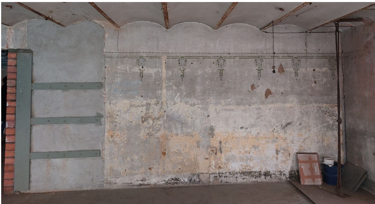
PA- Parament interior mitgera
