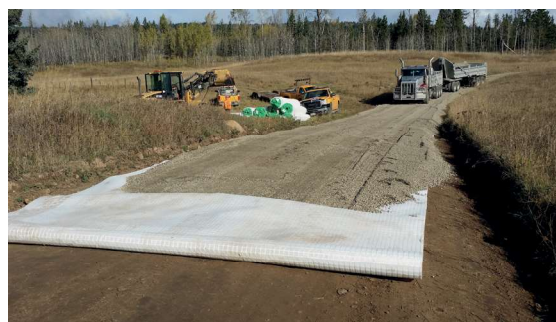
Figure 7: Combigrd® and Secugrid® installation
