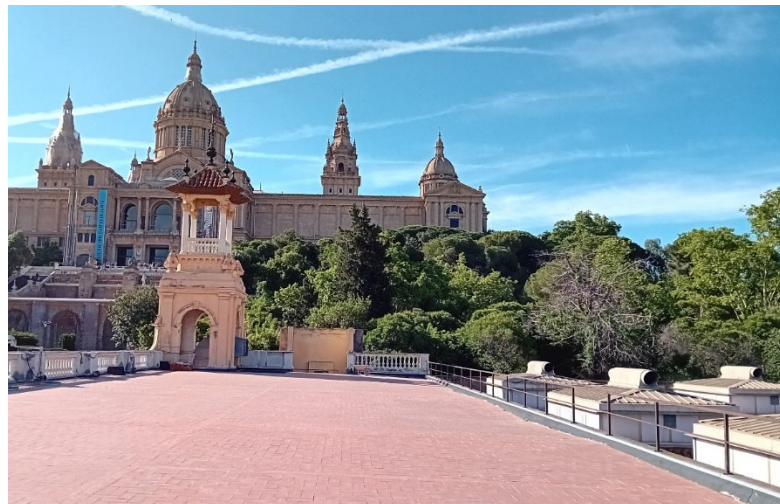
Roof and towers
