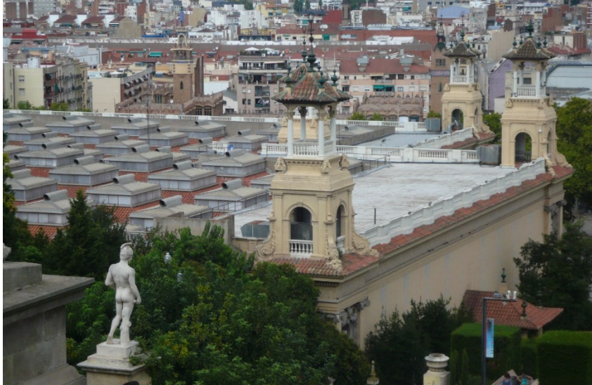
Roof and towers
