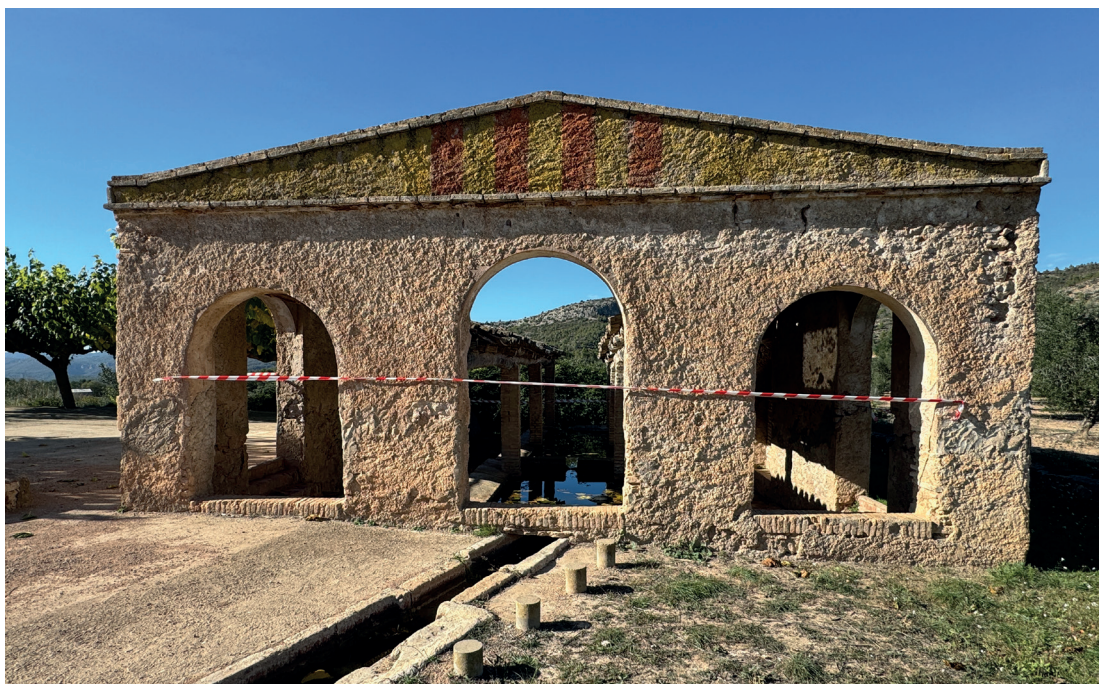
DF.2. Façana principal
