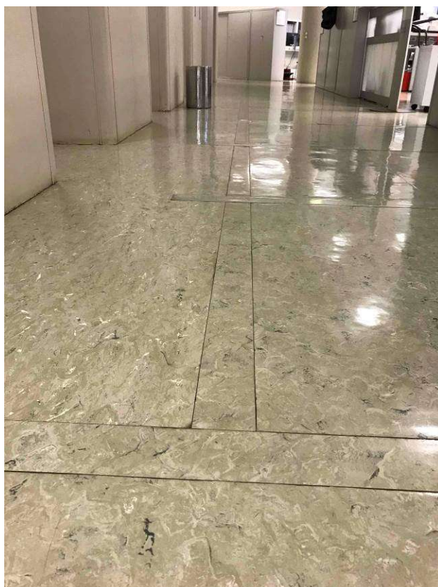
F12. Vista general interior
