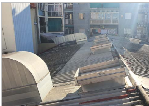
F09. Vista general coberta nau
