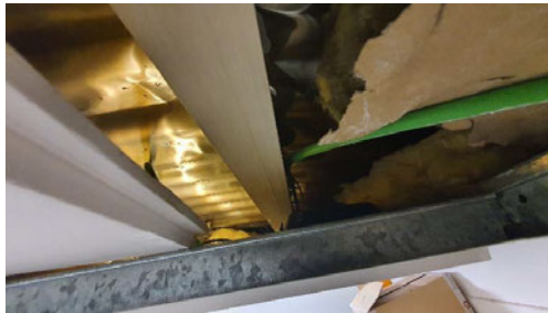
Interior del cel ras
