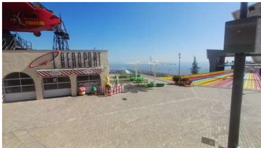
03 LOT 1 NIVELL 6 General accessos 3
