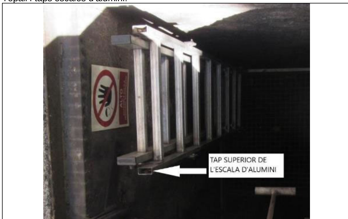
DETALL TAP SUPERIOR ESCALA ALUMINI
