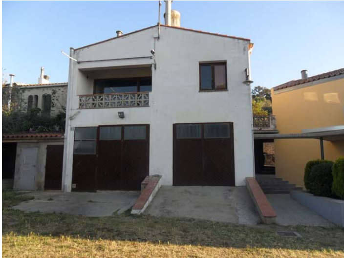
Detall façana principal
