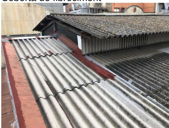
Coberta de fibrociment
