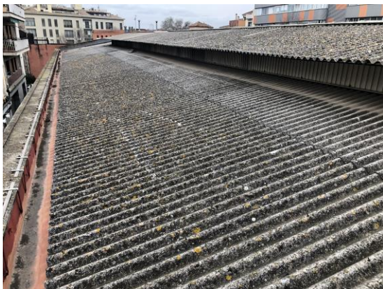
Coberta de fibrociment
