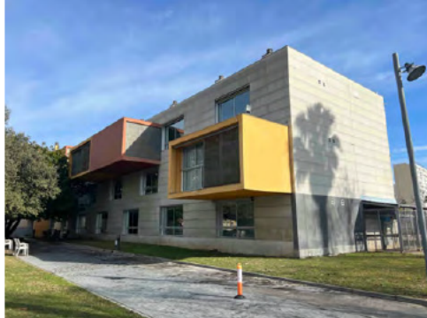
Vista general façana principal
