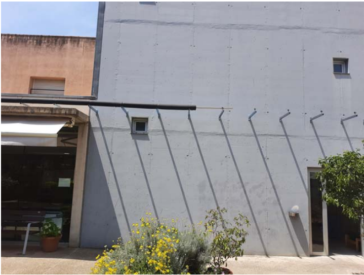
Detall 2 tram canonada a desmuntar
