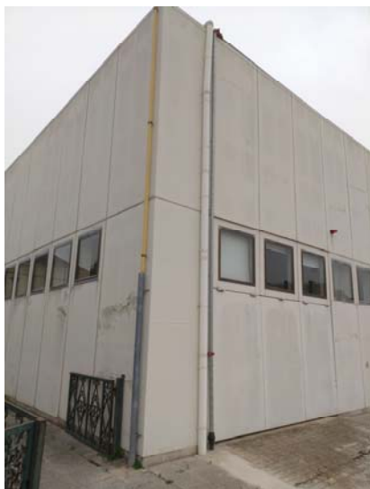
Exterior i interior porta basculant
