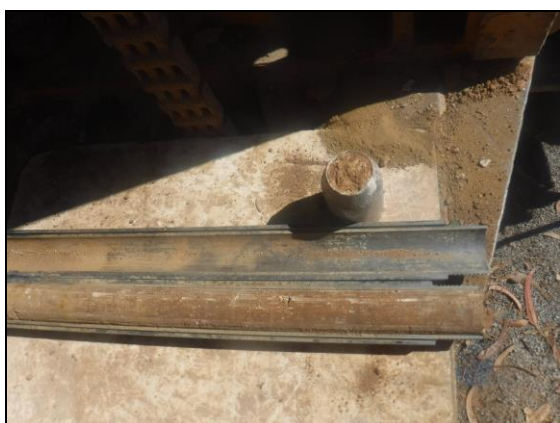
Foto 5: Sondeig S-2, SPT a 1,0 metre.
