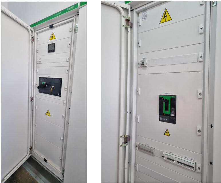
Detall portes quadre general BT
