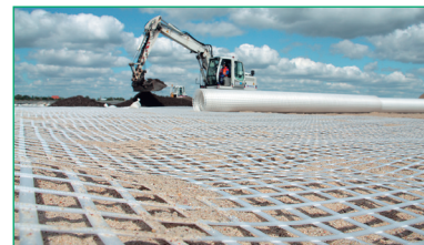
Figure 13 Secugrid® installation
