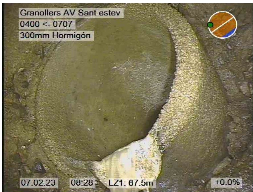
107.jpg, 00:08:58, 67.50m POZO FINAL CON 1 ACOMETIDA
