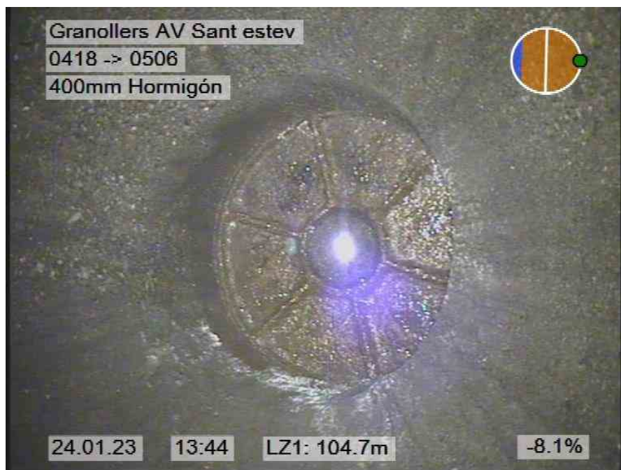
53.jpg, 00:10:43, 104.70m FINAL DE LA INSPECCION
