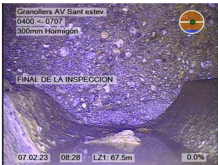
108.jpg, 00:09:17, 67.50m FINAL DE LA INSPECCION
