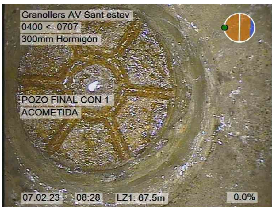
106.jpg, 00:08:58, 67.50m POZO FINAL CON 1 ACOMETIDA
