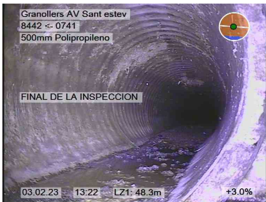
72.jpg, 00:06:54, 48.30m FINAL DE LA INSPECCION
