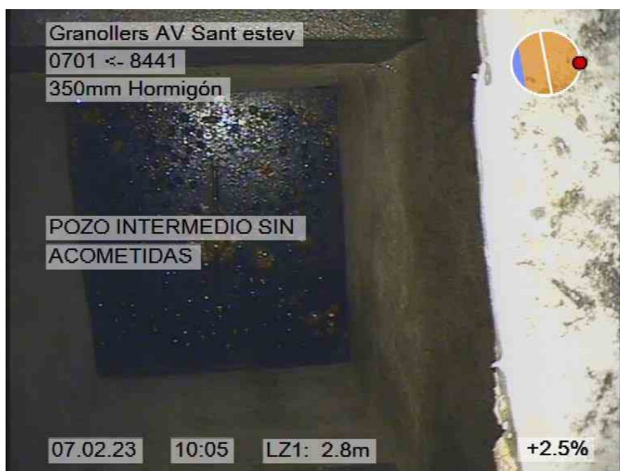
114.jpg, 00:00:46, 2.80m POZO INTERMEDIO SIN ACOMETIDAS
