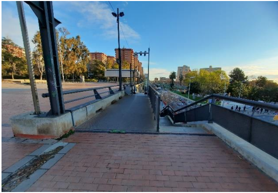
Coberta plana transitable
