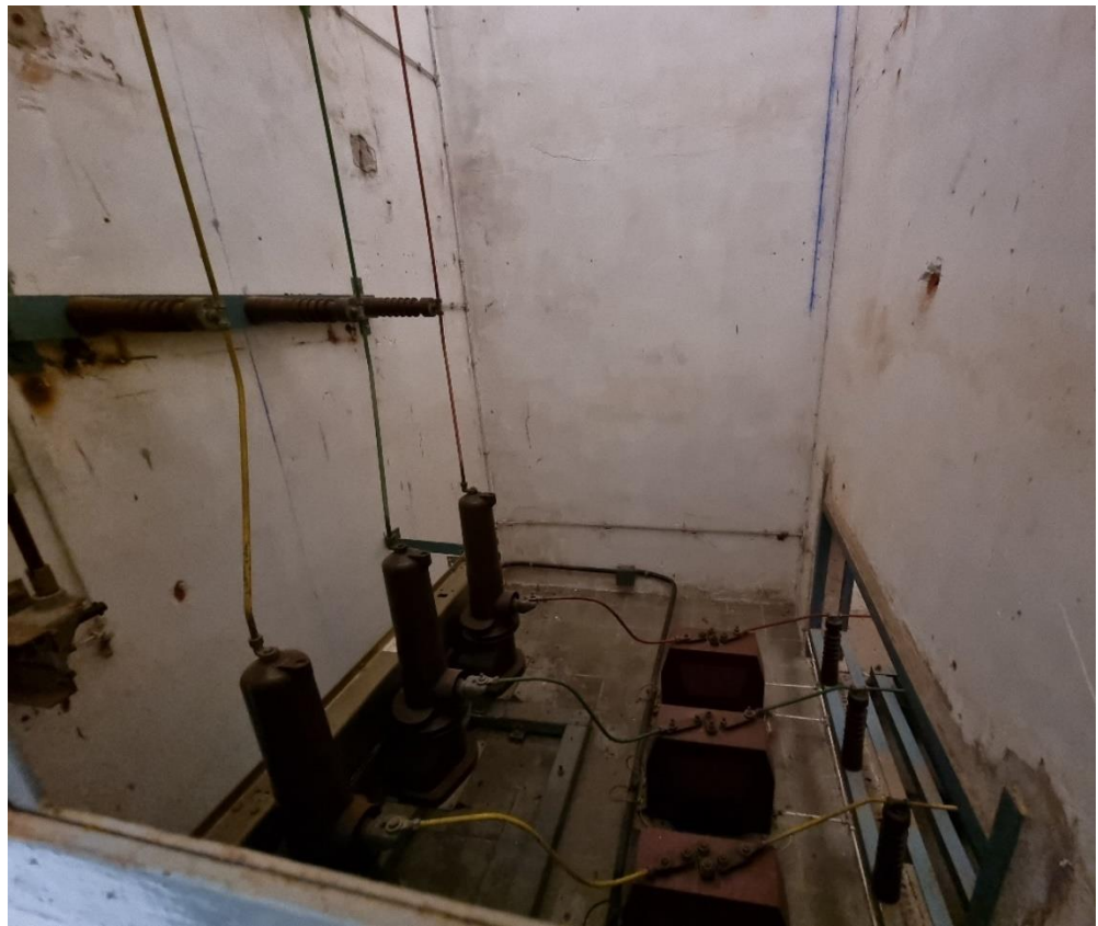
Interior CRM a reformar
