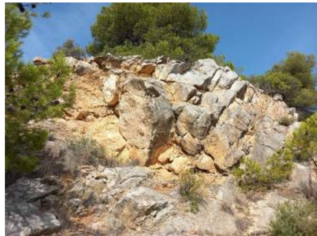
Figura 5. Masses potencialment inestables al talús PG01TA13D
