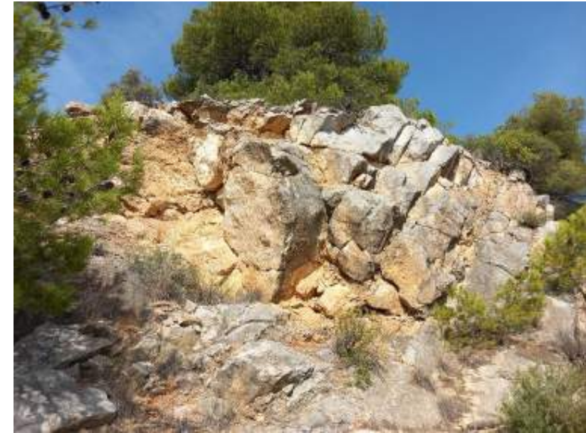
Figura 10. Masses potencialment inestables al talús PG01TA13D
