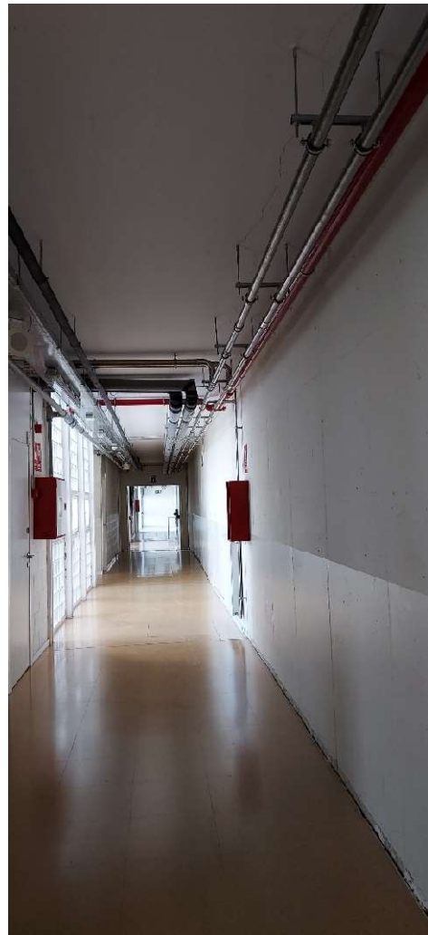
Passadis principal Soterrani
