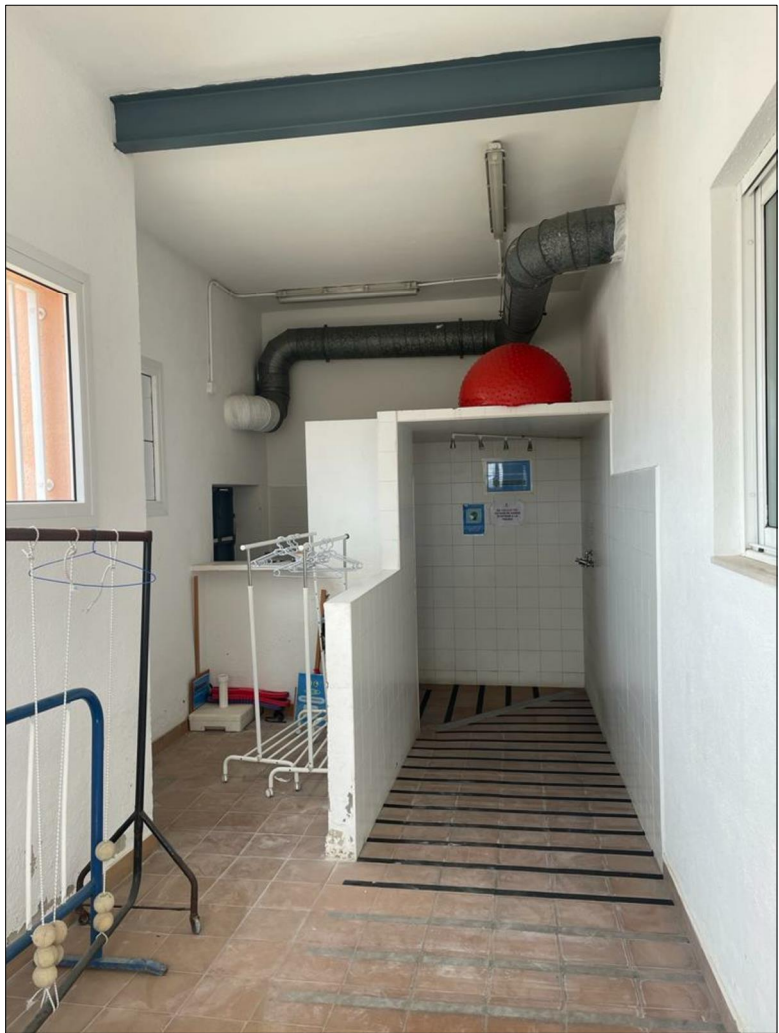
sostre a enderrocar rampa a refer
