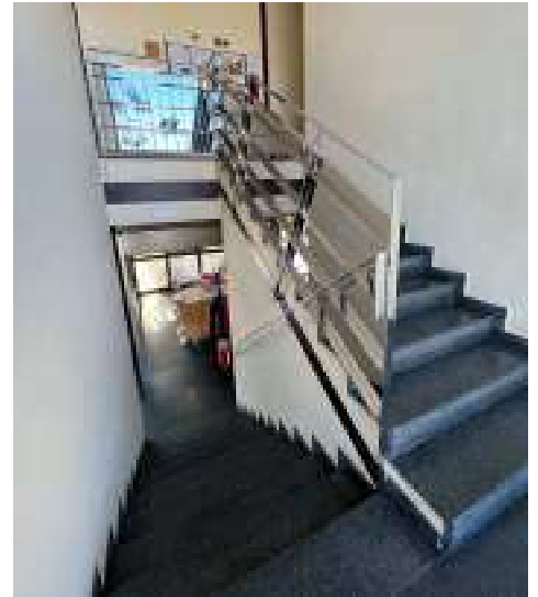
Escala interior existent.
