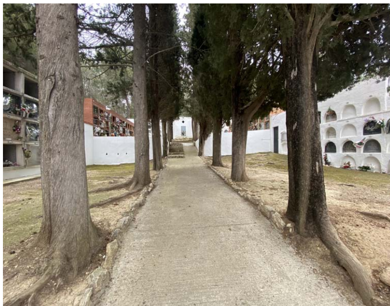
Passadís central a rehabilitar.
