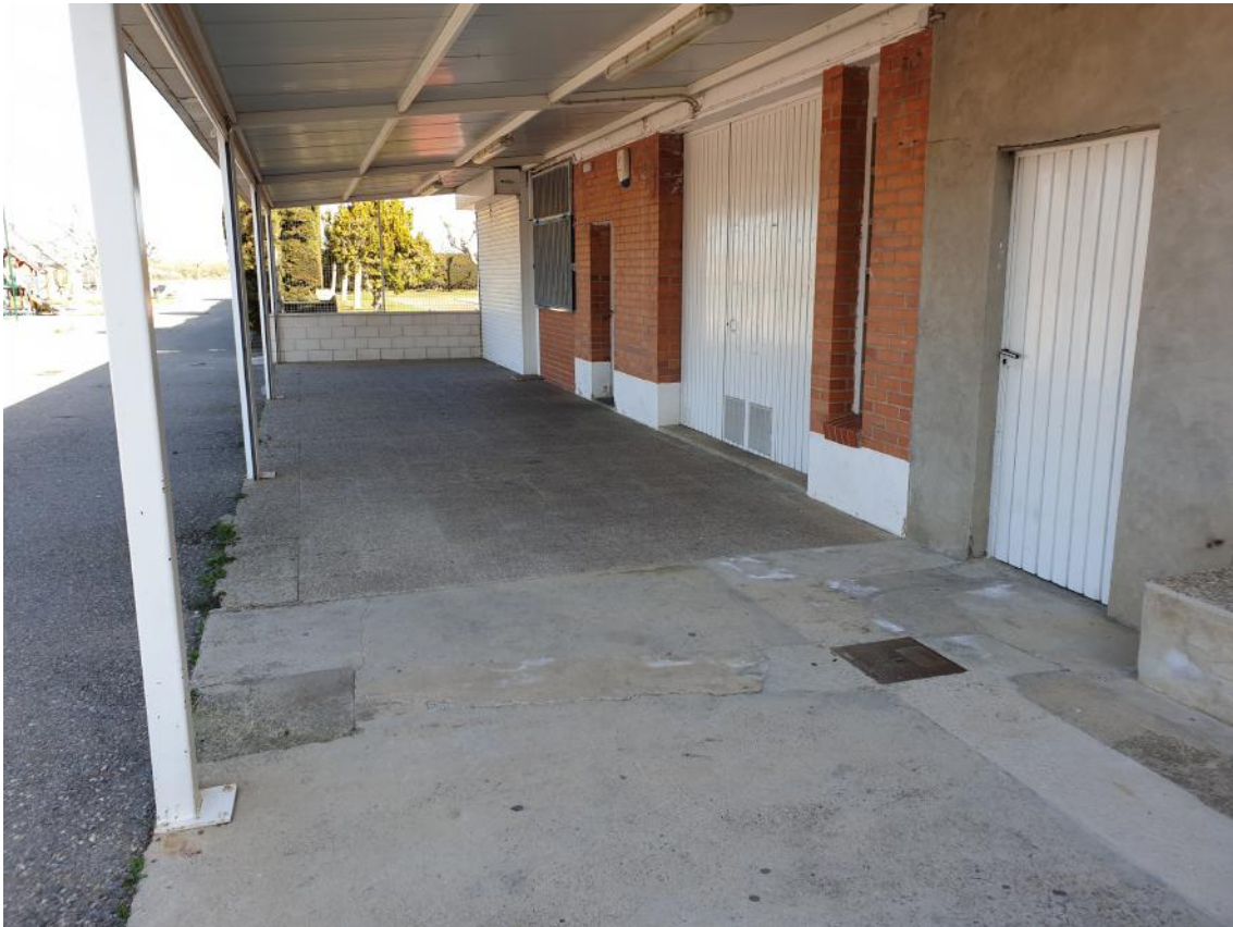
Porxo exterior – façana principal
